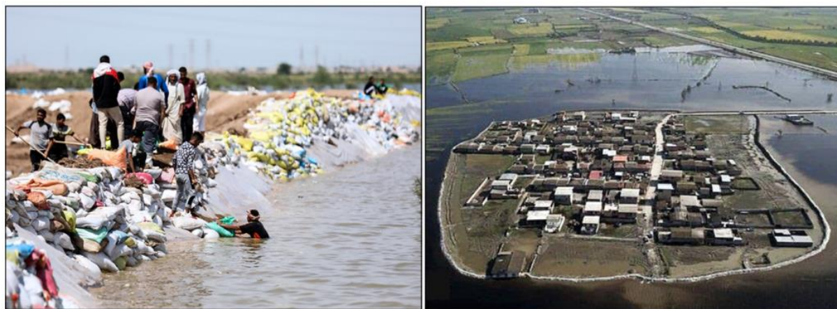
Fig. 10. Images showing the construction of a flood wall by locals.
